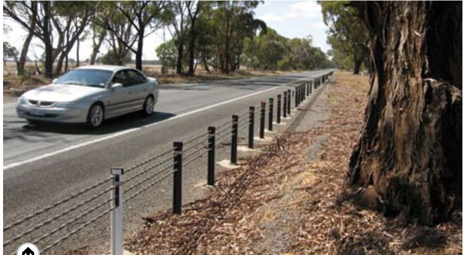
Run-off road crashes account for around 139 deaths every year. Installing safety barriers at the side of the road means that cars do not collide with roadside vegetation
