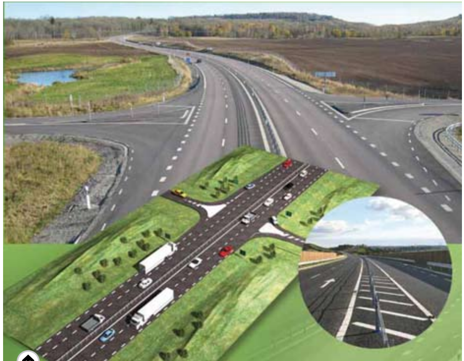
The above shows a Type 2 carriageway, which consists of two lanes in each direction, separated by wire-rope safety barriers
